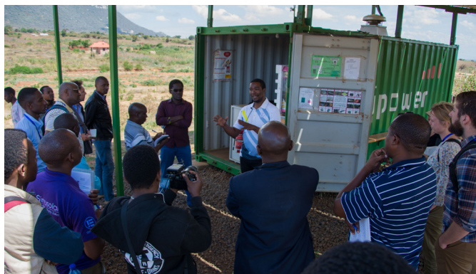
Khalfan Hussein explains Rafiki Power's mini-grid system in Chang'ombe and Dongo
